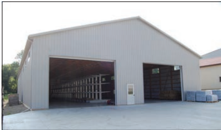
2018 Warehouse for Conventional Lumber
