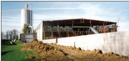
2000 New Warehouse Addition
